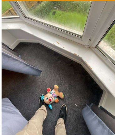
07-10-2023 13:39 / Bedroom Windows Sills / J01ezfqa2
