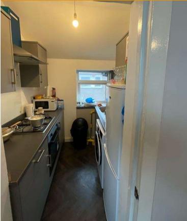
07-10-2023 13:35 / Kitchen Walls Ceilings / W3x70zr47
